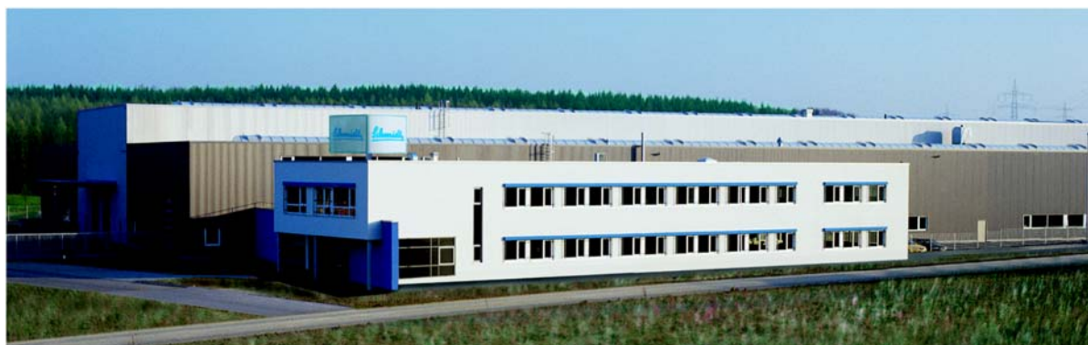
First class technology from an up-to-date plant
